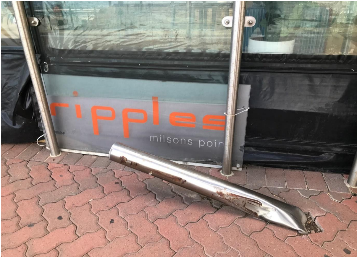
Photos of damage caused by large vehicles accessing Olympic Boulevard to get into and out of Luna Park.
